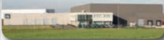
BENELUX LOGISTIC CENTER
